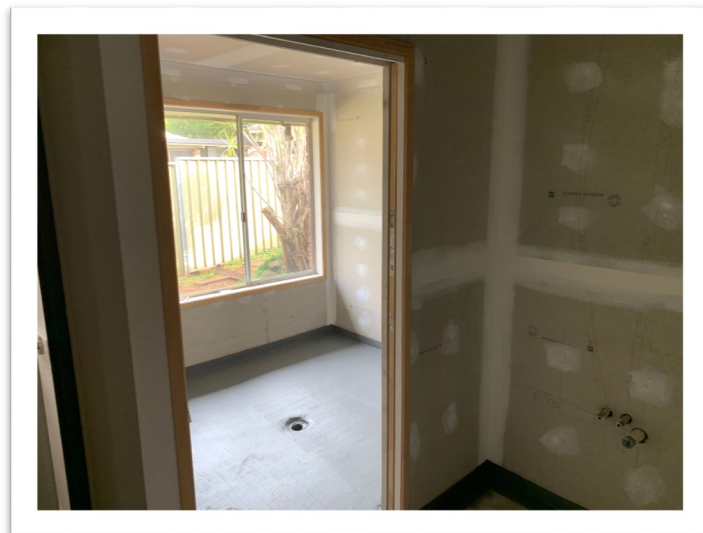
New Bathroom at the Respite House
